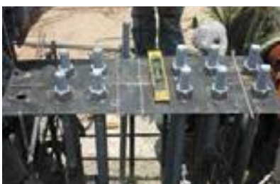
Setting up Anchor Bolt
