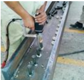
Shear stud connection
